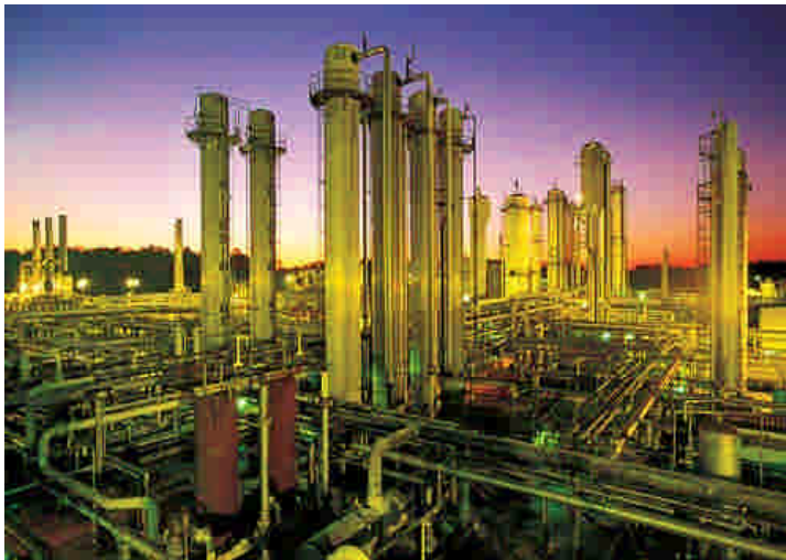
Typical Gas Plant Site
